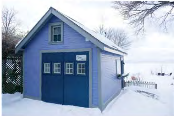
The original garage door was reconstructed as the back wall, with salvaged windows. One of the windows looks into the tiny but efficient kitchen; the other three windows are in the bathroom.
