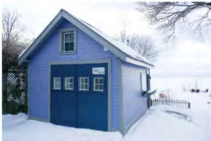
The original garage door was reconstructed as the back wall, with salvaged windows. One of the windows looks into the tiny but efficient kitchen; the other three windows are in the bathroom.
